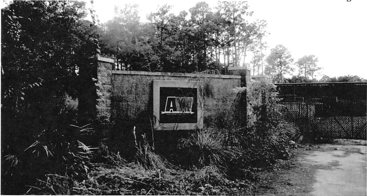
Violation: Unpermitted wall and signs. The signs on the property are in violation of the conditions of PUD Ord. 2009-286-E. Addressed assigned: 11310 Dunn Creek Road.
