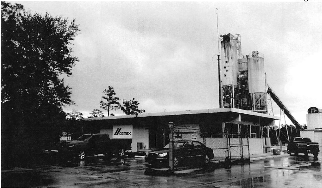
Example of concrete batch mixing plant: 750 Eastport Road
