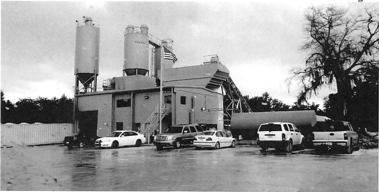
Example of concrete batch mixing plant in the area: 1220 Eastport Road
