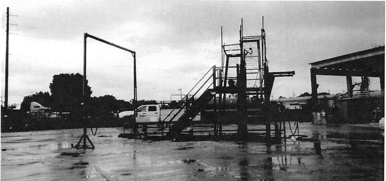
Example of wash down area for trucks: 1220 Eastport Road
